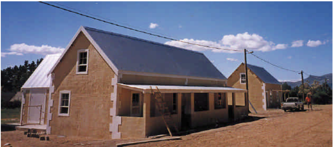
Photo 3: Example of stoep with partially open end walls supported by plastered columns.
